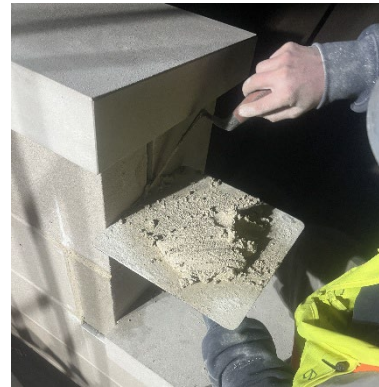
Figure 7: Masonry Facade Restoration
