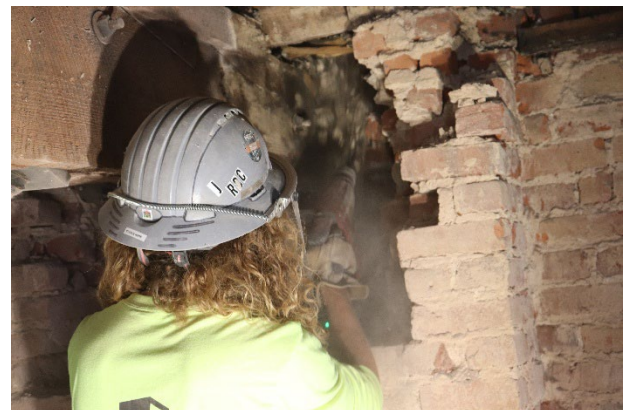
Figure 4: Demolition of the deteriorated masonry
