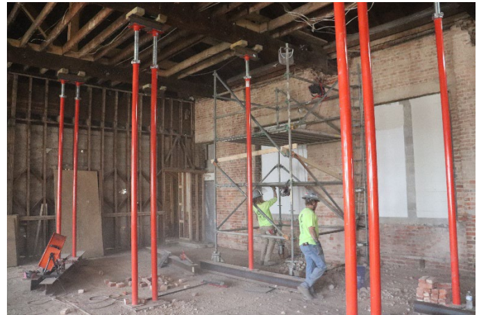
Figure 3: Shoring holding the roof aloft while the team works
