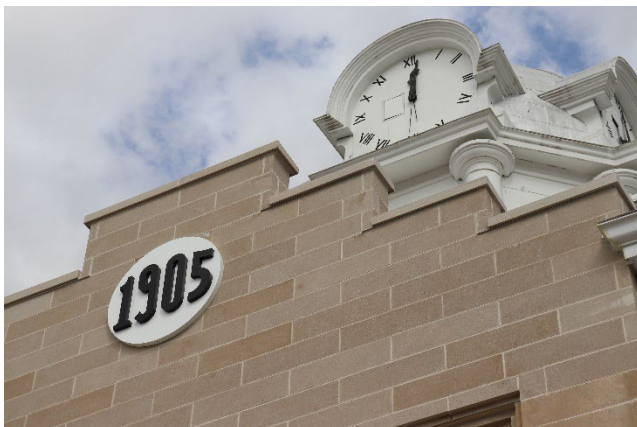
Figure 8: Newly restored facade
