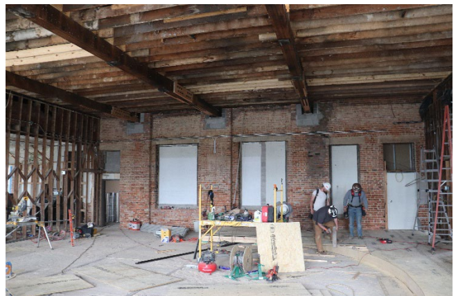
Figure 9: Fully complete truss system
