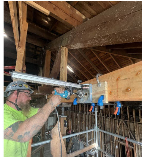
Figure 5: Drilling holes in truss to install additional support system
