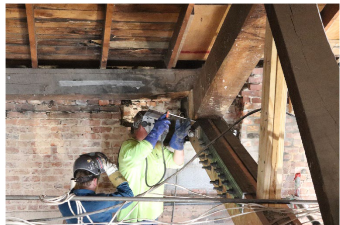
Figure 6: Installation of turnbuckle style support system
